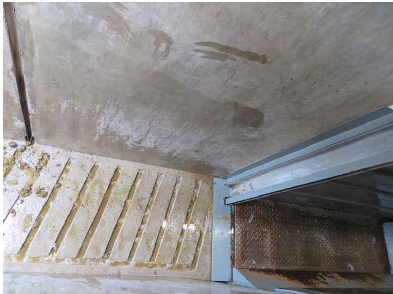
Figure 2: The transfer from the driving corridor to the shoot box has a grey, metal crosswise stripe that halt the horses while walking.
