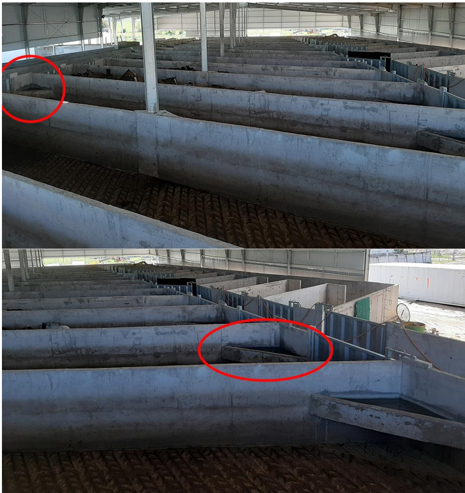
Figure 6: A fishbone-shaped waiting stall and high, equally close side walls in the driving passageways.
